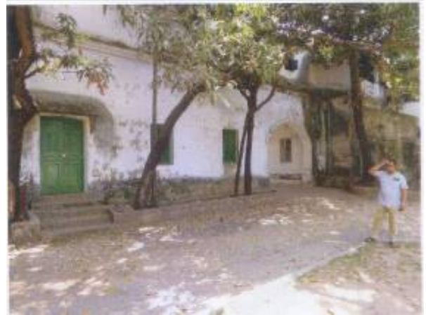
Fig: Front view of building
