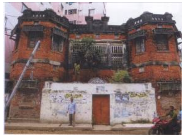
Fig: Front View of building
