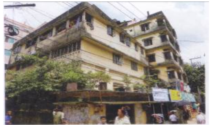
Fig: Front View of building
