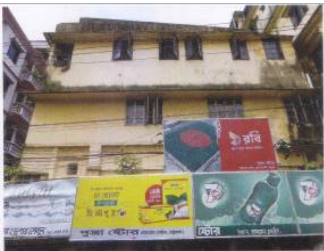
Fig: Front view of building
