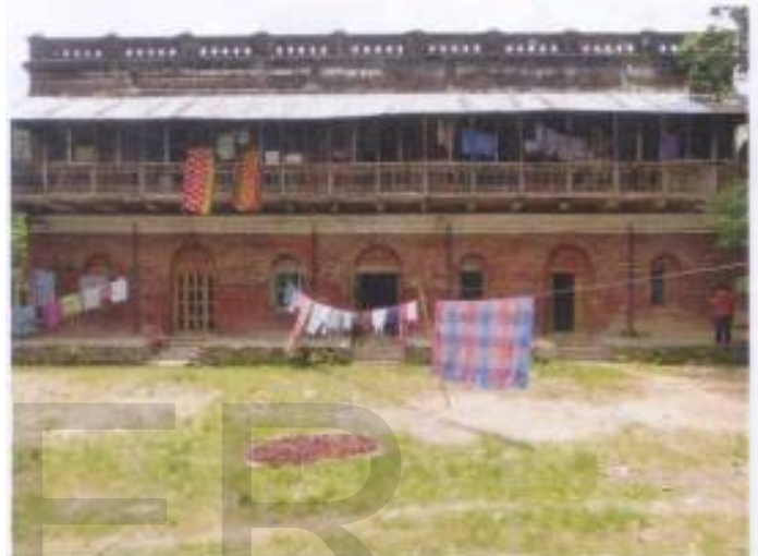
Fig: Front view of building
